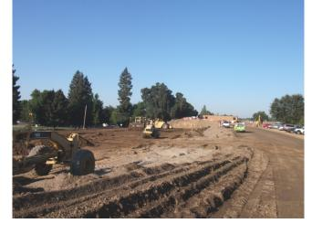
subgrade cap from Station 71+50 to 77+00 required over excavation of 18" in order to achieve a stable subgrade because of overly moist in situ soil conditions. Backfill material for the subgrade cap was from two sources, offsite from Aspen 3 and from the degrade of the levee west of Station 73+00.
