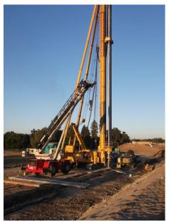
On the 31st of August Drill Rig #1 lost a cutting head at - 59' from the work pad and was unable to push through it. This required that a section of wall be added waterside parallel with and adjacent to the original. The parallel wall is 5 elements long with the outer two at a skew to tie back into the design wall, ensuring continuity. The work for this parallel wall was completed on the 6th and 7th of September.
